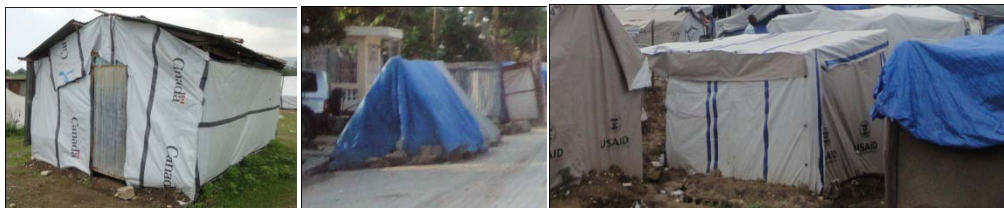
Examples of shelters build with plastic sheeting. Left and right: “box frame”; centre: “A frame”
