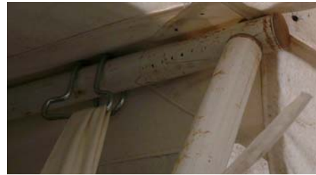
Detail of ridge fixings showing wire hooks which might cause canvas to fail over time.
