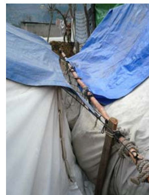
Adaptation: fixing guy ropes to a pole and beam rather than to pegs. This saves space and can help in hard ground where it may be difficult to fix multiple pegs.
