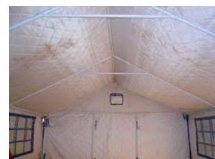
Interior of frame tent showing partial trusses.
